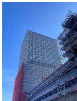
Chantier Tilia Tower
