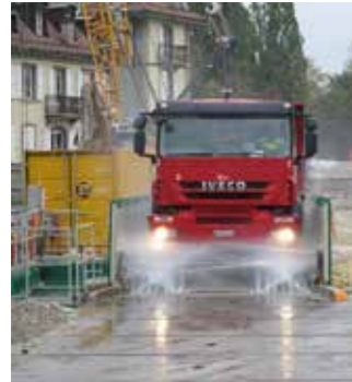
CIO site - truck cleanings
