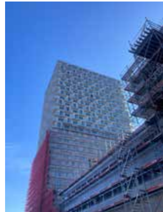
Tilia Tower construction site
