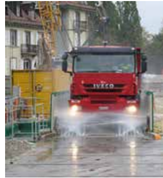
CIO site - truck cleanings
