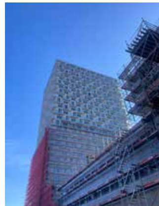
Chantier Tilia Tower
